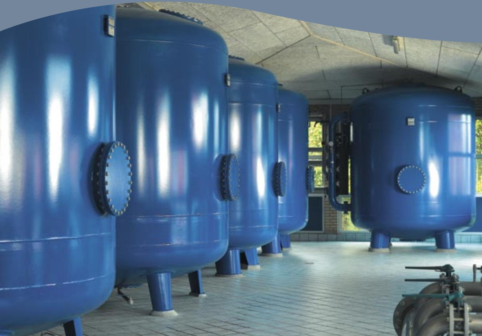
*Reduction of iron, manganese, aggressive carbon dioxide, and ammonium in waterworks. The solution comprises 5 x TFB 75 connected in parallel, blower, and rinse pump. Flow rate: 265 m<sup>3</sup>/h. The colour of the tanks is custom-made.*
