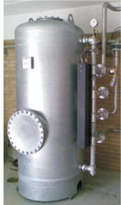
*Arsenic removal by means of adsorption in waterworks. The solution comprises an automatic pressure filter type NSB 170 installed after open filters. Flow rate: 12 m<sup>3</sup>/h.*
