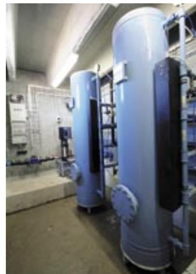
*A great many consumers are situated so that connection to a large, municipal waterworks is not practical or desirable. The technical solution will of course be based on the same principles as the large water supplies. A pressure filter type NSB is ideal for small and medium drinking water supplies.*
