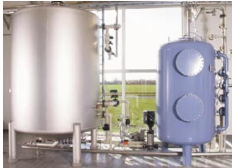
Degassing of dissolved gases such as aggressive carbon dioxide, methane, and hydrogen sulphide is a precondition of optimum filtration. Photo: degassing and pressure filtration in brewery.
