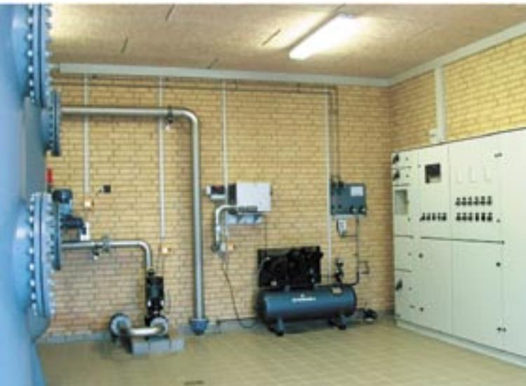
Complete water treatment solution comprising a pressure filter and technical equipment for oxidation and backwashing.
