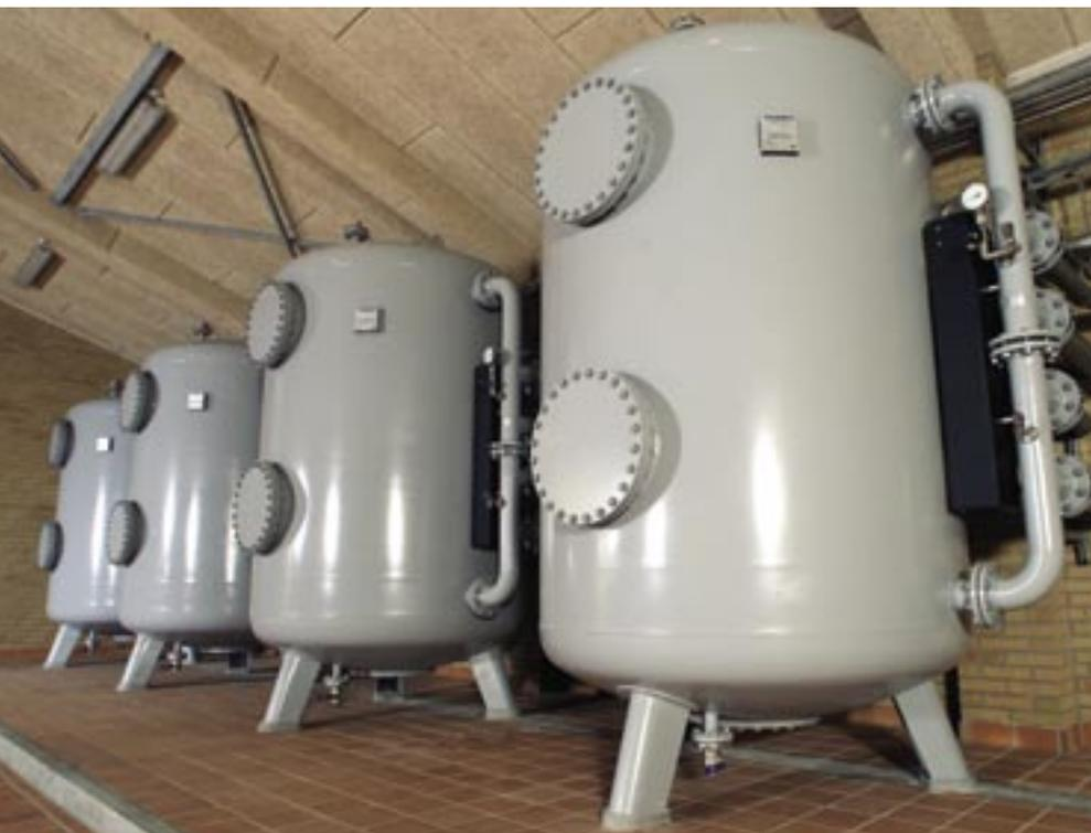
*Removal of iron, manganese, and ammonium in waterworks. Flow rate: 2 x 35 m<sup>3</sup>/h.*
