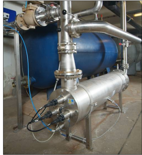
UV system type Spektron 70 with a flow rate of 108 m 3 /h. The system is installed in a dairy.
